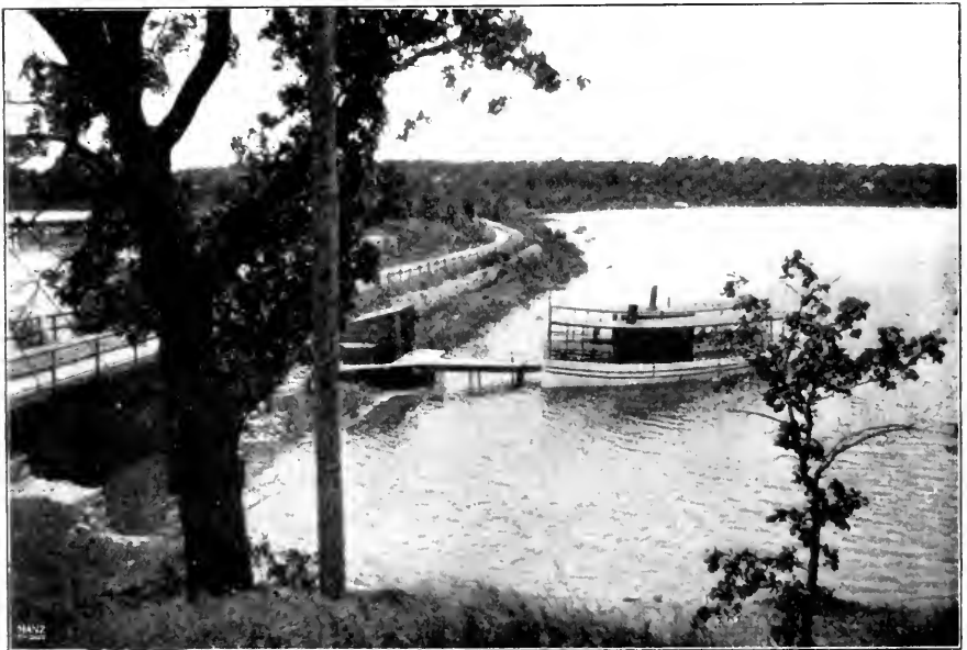
OKOBOJI BRIDGE AND GRADE LOOKING NORTH.
