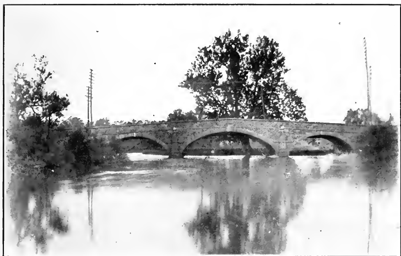
THE LANCASTER PIKE BRIDGE, BUILT IN 1802.
