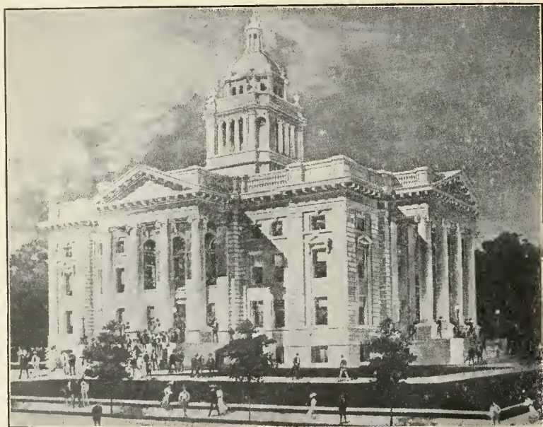
New Court House at Jasper, 1910. (Under Construction, 1909-1910.)
