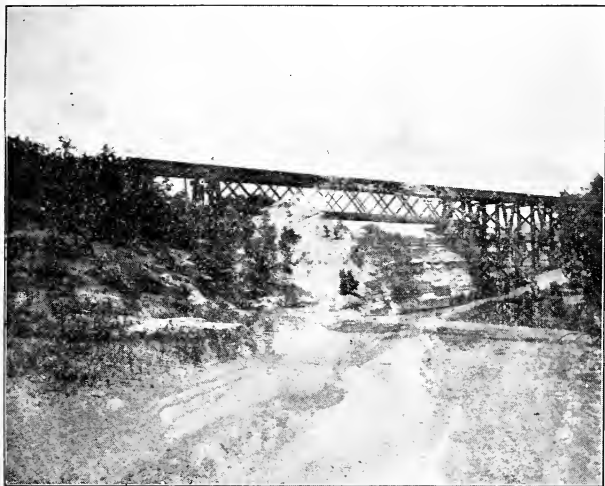
THE BRAZOS RIVER BRIDGE
