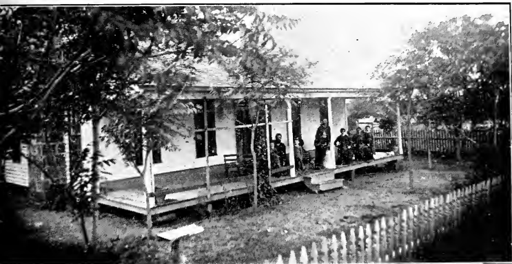
W. C. MCGOUGH'S RESIDENCE
