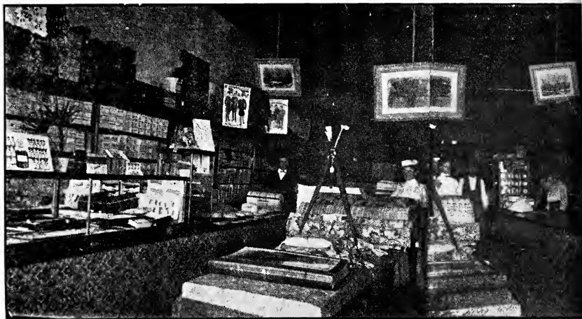
INTERIOR VIEW OF GEORG
