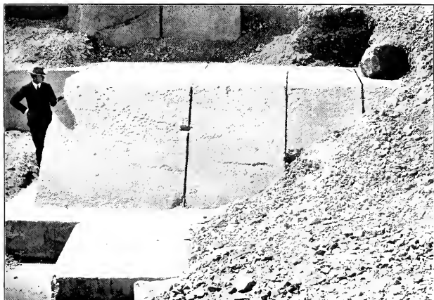
FIG. 66 —CASING BLOCKS AT THE BASE OF THE GREAT PYRAMID JOINTS OTHERWISE UNDISCERNIBLE INDICATED BY CHARCOAL LINES.
