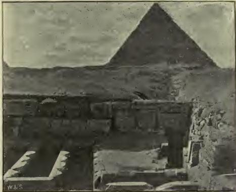
FIG. 30.—West side of granite temple, showing passages and causeway leading askew up to temple of second pyramid.
