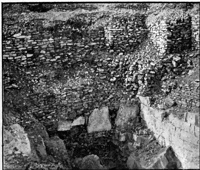
Fig. 53.—Rubble walls and chips forming the mass of the pyramid. At the right is the top of the chamber masonry.
