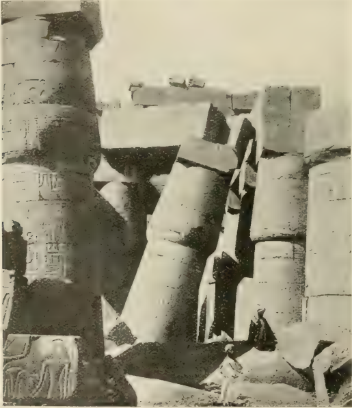
FIG. 8.—Great hall of columns. Karnak.
