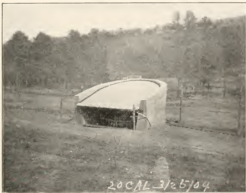
HORSE-SHOE TYPE OF WHEEL MILL.
