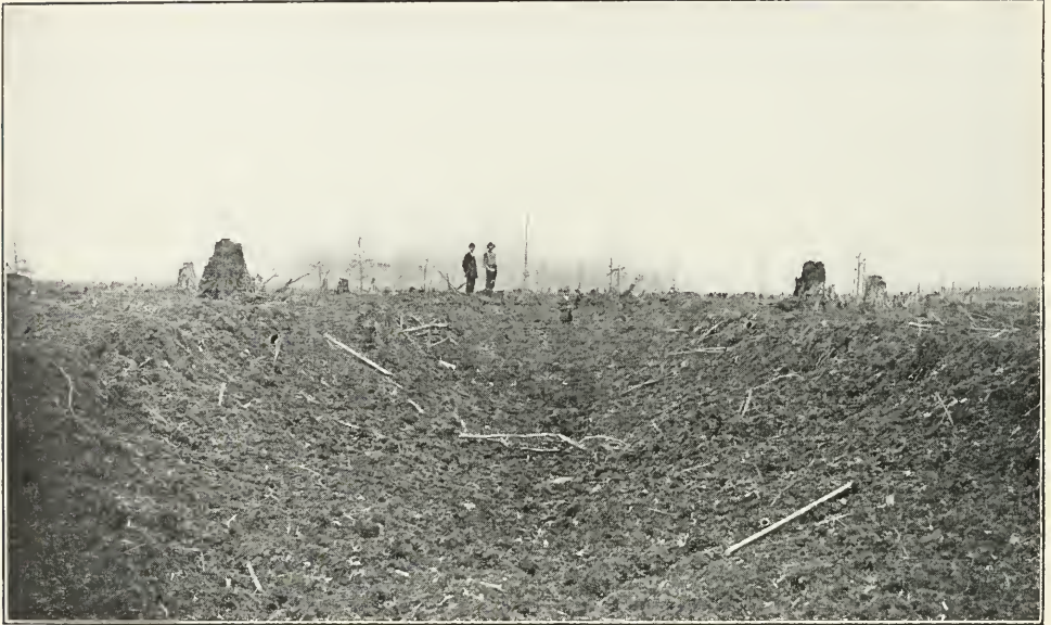
BLASTING A DITCH—AFTER THE BLAST.
