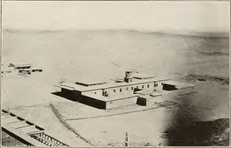
ADMINISTRATION HOUSE OFICINA "DELAWARE" VIEWED FROM TOP OF OLD MAQUINA.
