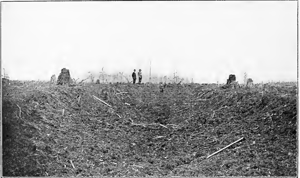
BLASTING A DITCH—AFTER THE BLAST.
