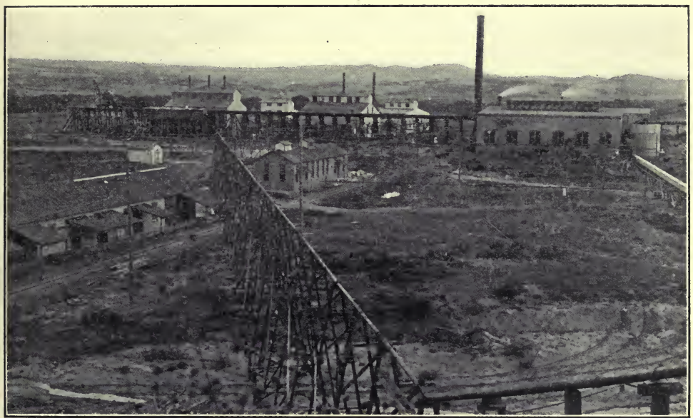
POWER HOUSE AND ACID PLANT, LOUVIERS, COLORADO.
