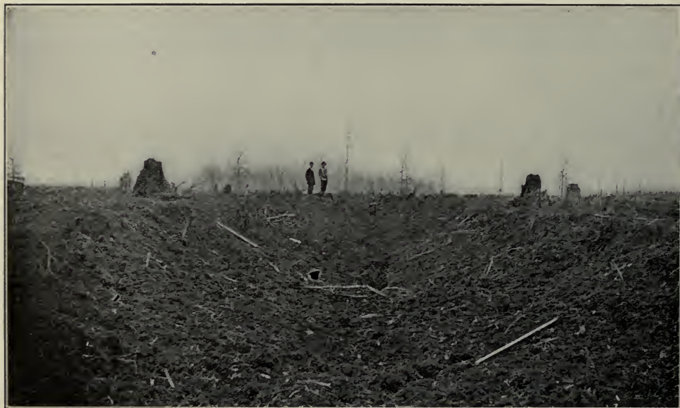
BLASTING A DITCH—AFTER THE BLAST.
