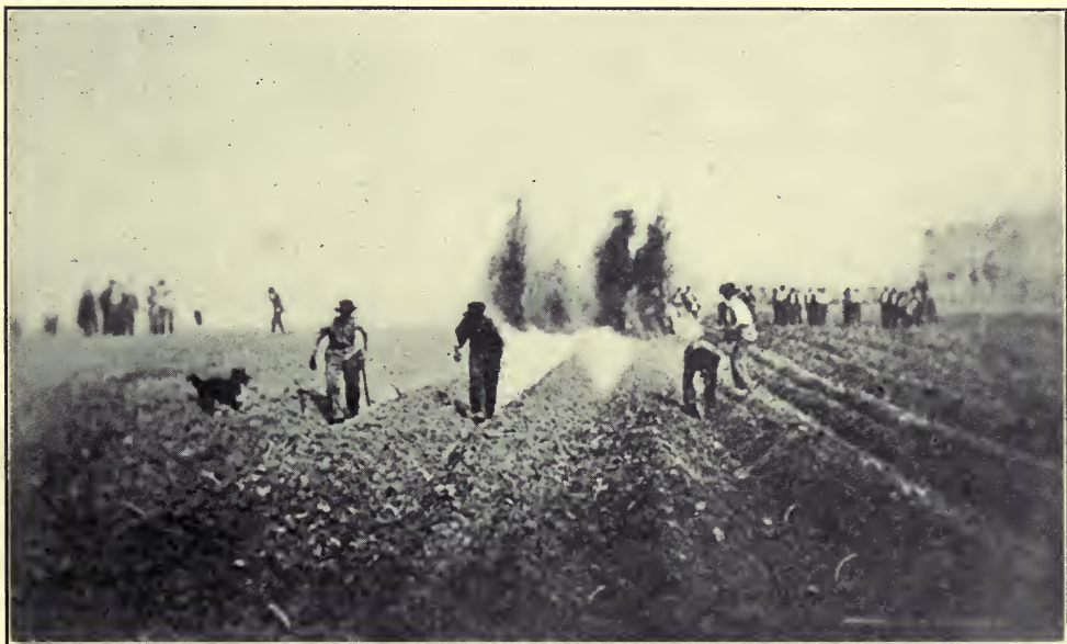
SUBSOILING WITH DYNAMITE—LIGHTING THE FUSE.
