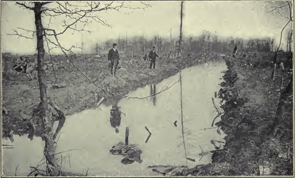
BLASTING A DITCH—AFTER THE WATER HAS BEEN LET IN.
