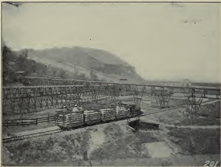
PLANT TRANSPORTATION OF DYNAMITE.
