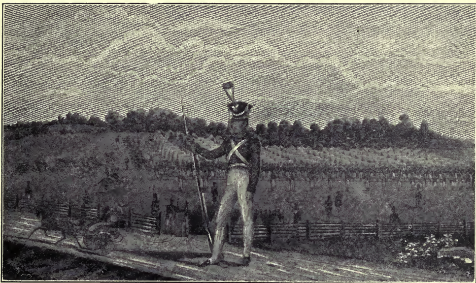
AMERICAN TROOPS GUARDING DU PONT POWDER WORKS ON THE BRANDYWINE, NEAR WILMINGTON, DEL., DURING THE WAR OF 1812.
