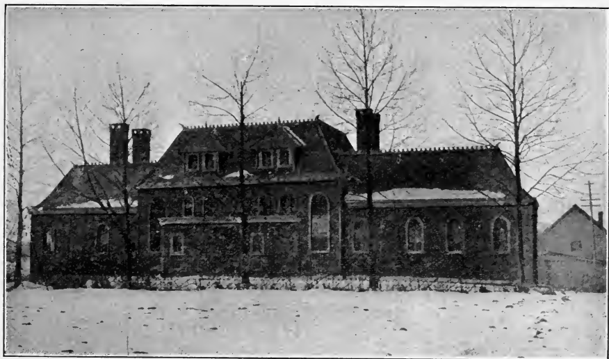
SECOND OFFICE OF E. I. DU PONT DE NEMOURS AND CO.—ANOTHER VIEW.
