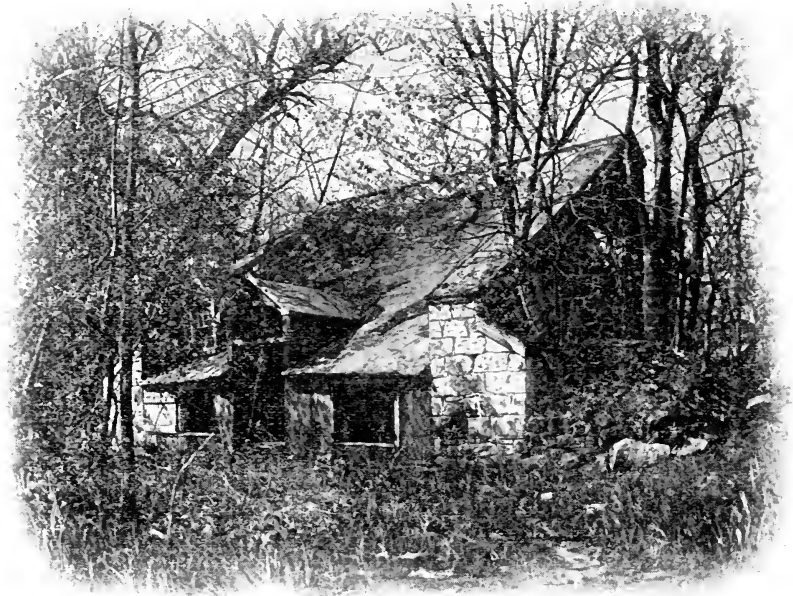
FIRST DU PONT POWDER MILL ERECTED ON THE BRANDYWINE IN 1802.
