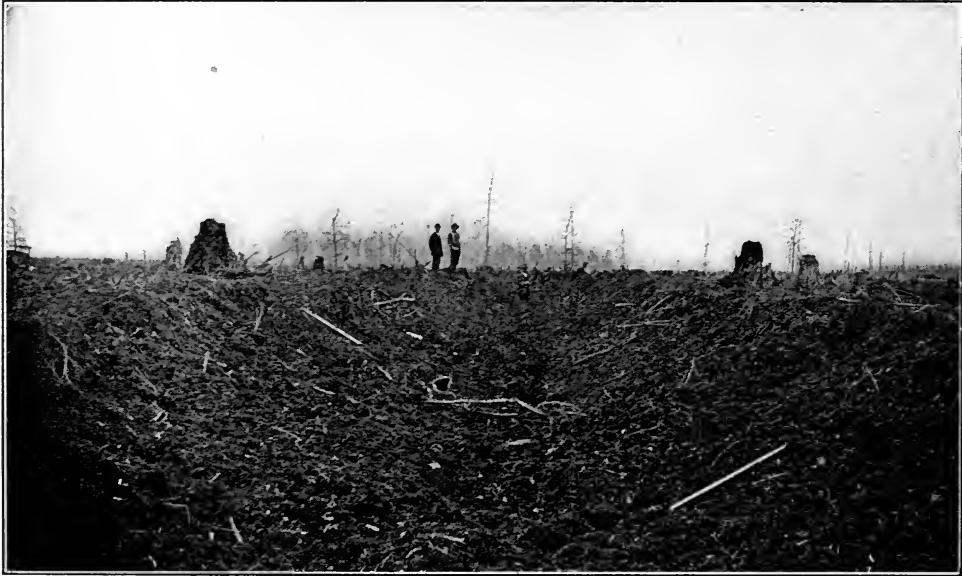
BLASTING A DITCH—AFTER THE BLAST.
