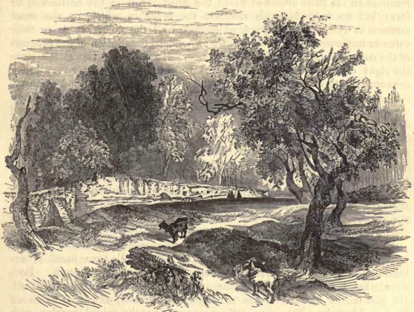
Hougoumont—Exterior of Garden Wall.
