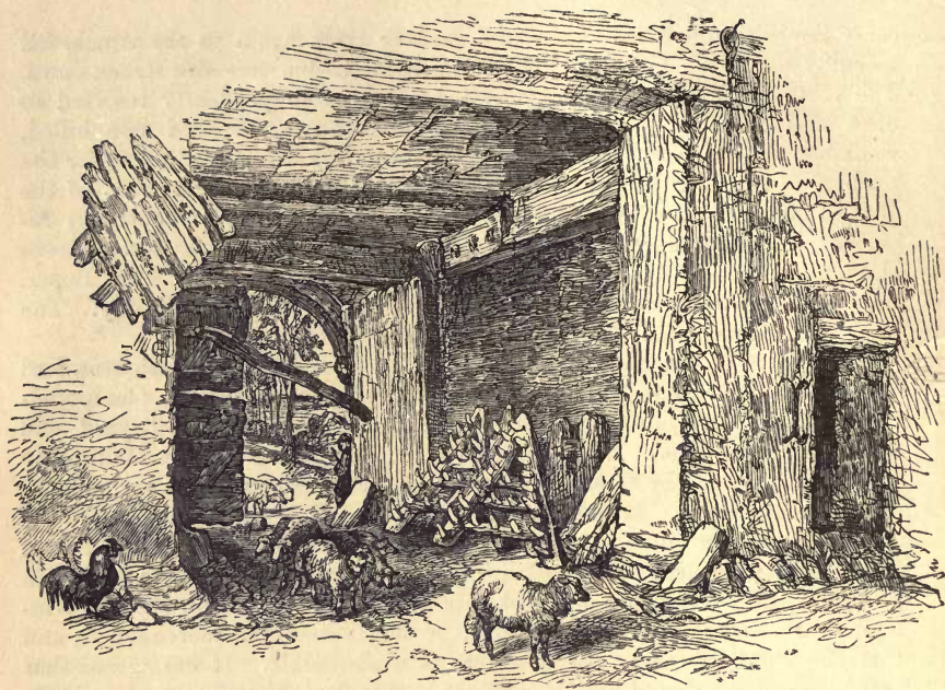
Hougoumont—Gateway of Farm-Yard, from the Interior.
