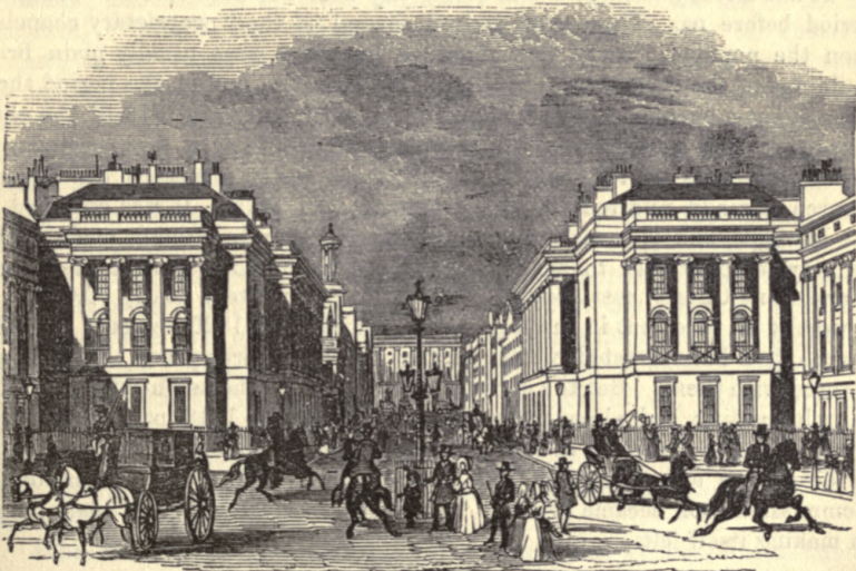
Waterloo Place, leading toward Regent-street.
