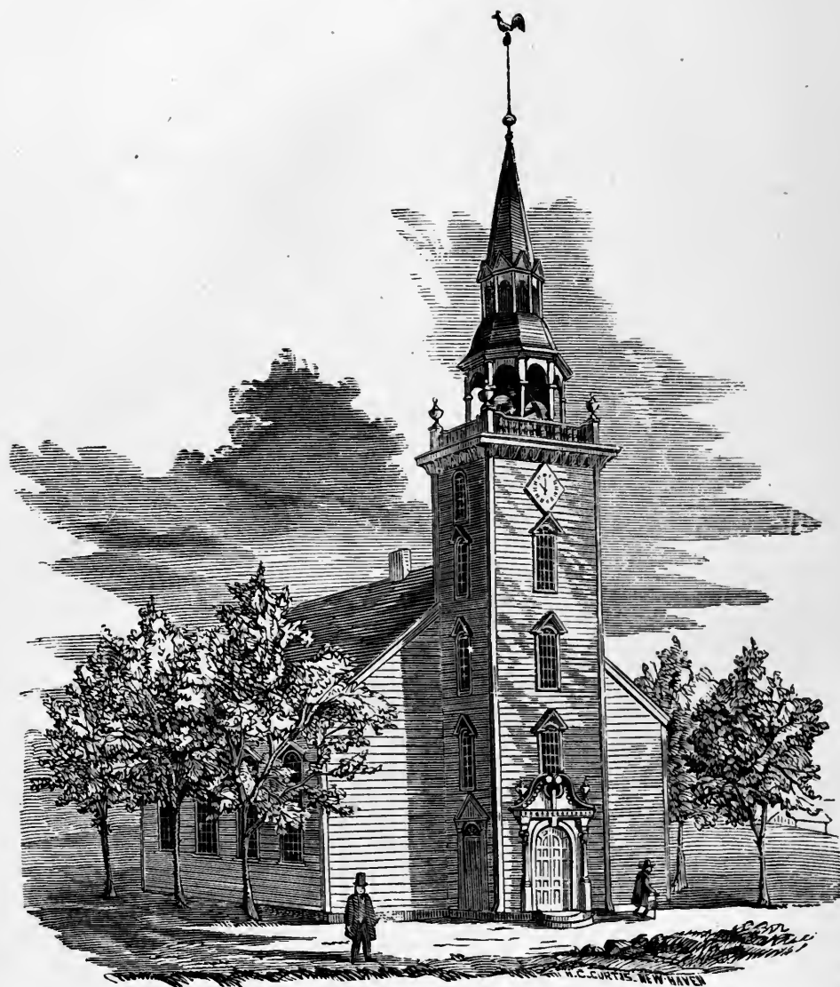
CHRIST CHURCH, STRATFORD, Erected in 1743, demolished in 1858.
