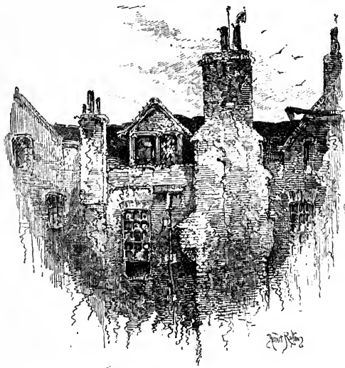
Chimneys facing the Slough Road.
