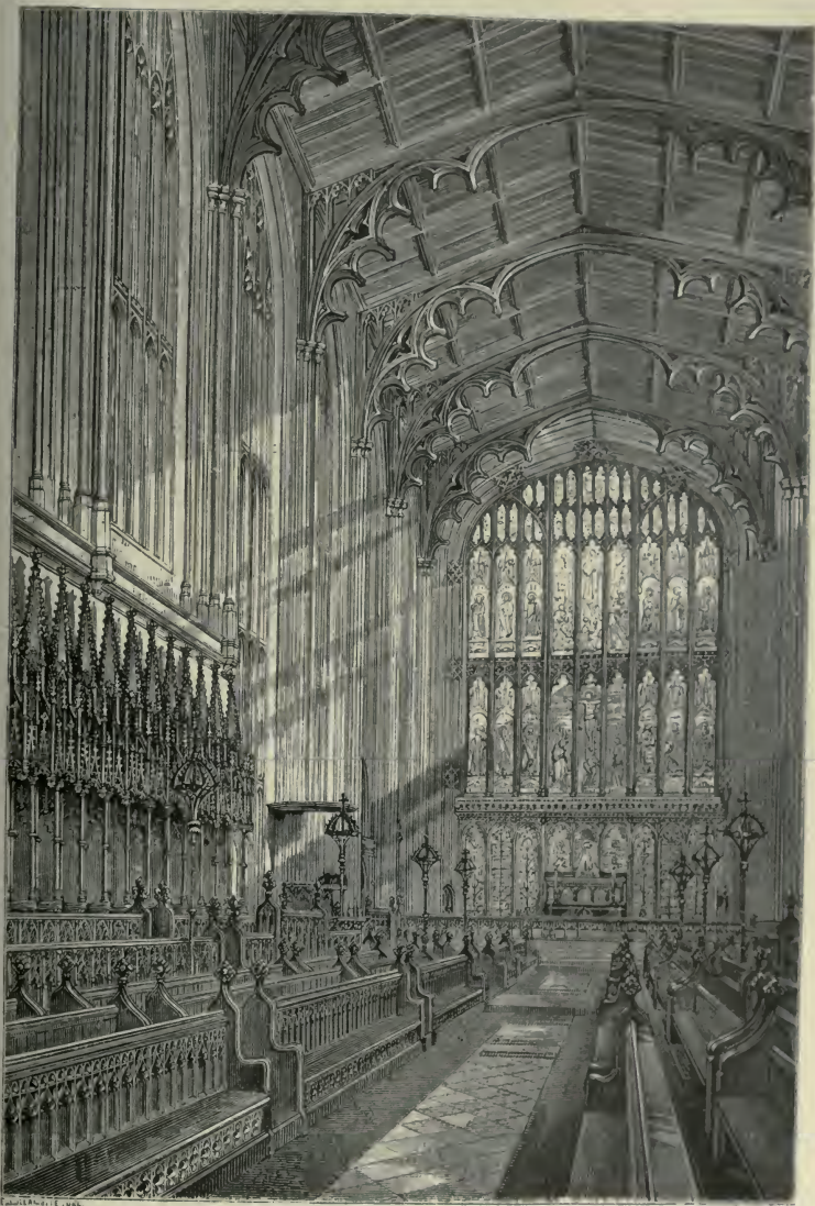
INTERIOR OF THE CHAPEL.
