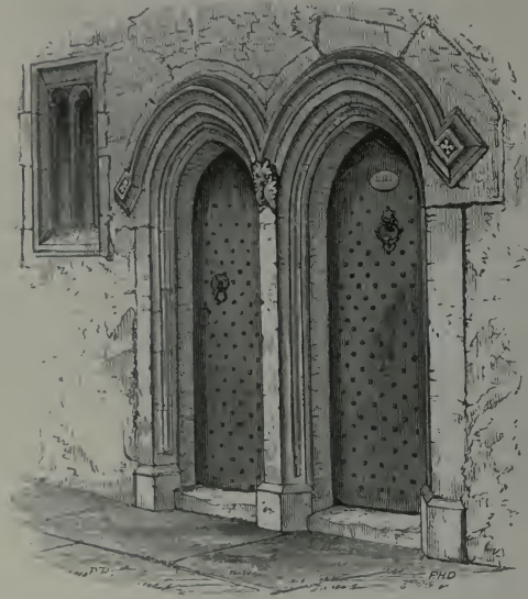
Double Doorway in the North Walk of the Cloister.
