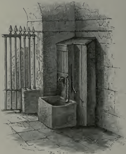
Pump in the Cloister.
