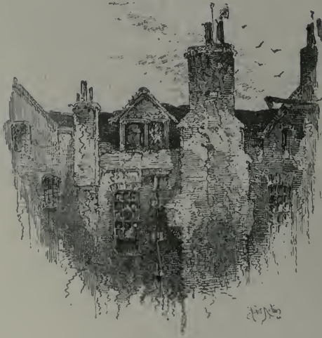
Chimneys facing the Slough Road.
