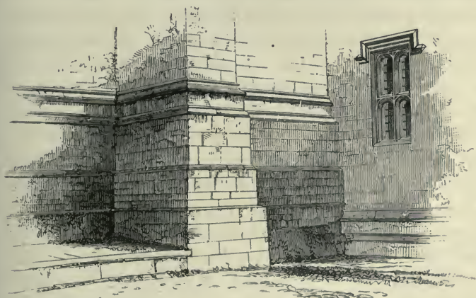
Buttress, and North Wall of the Ante-Chapel.
