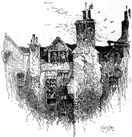
Chimneys facing the Slough Road.
