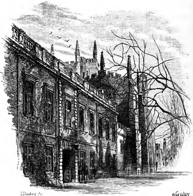
Exterior of the Upper School.
