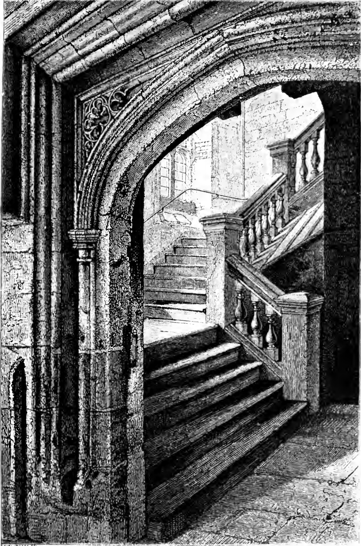
STAIRCASE TO THE CHAPEL AND UPPER SHELTER
