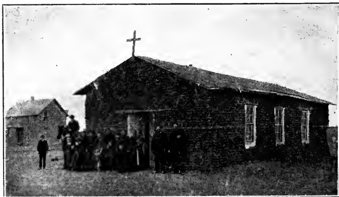
Sod houses and sod churches were not uncommon in the early days of Kansas and Nebraska. The above engraving is from a photo of a sod Lutheran church in Nebraska.
