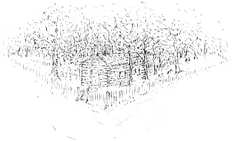
FIRST CHURCH BUILDING. Erected 1769. (Drawn from Description.)
