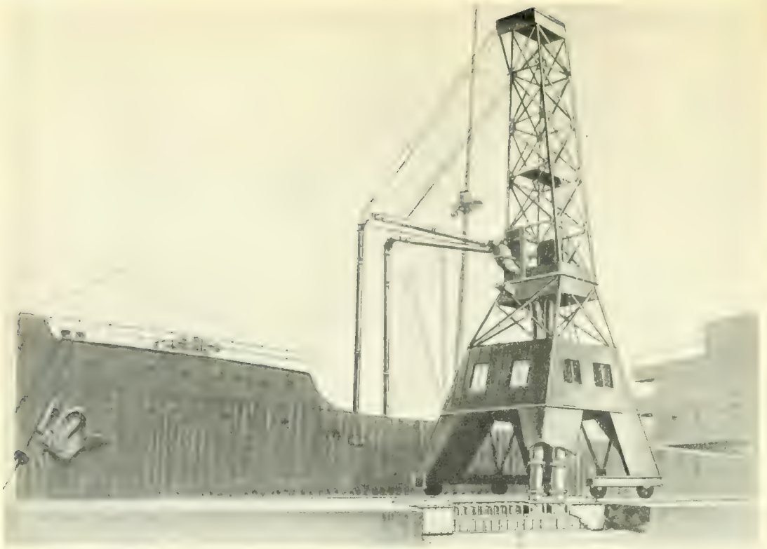
FIG. 52.—Pneumatic Unloading Plant.
