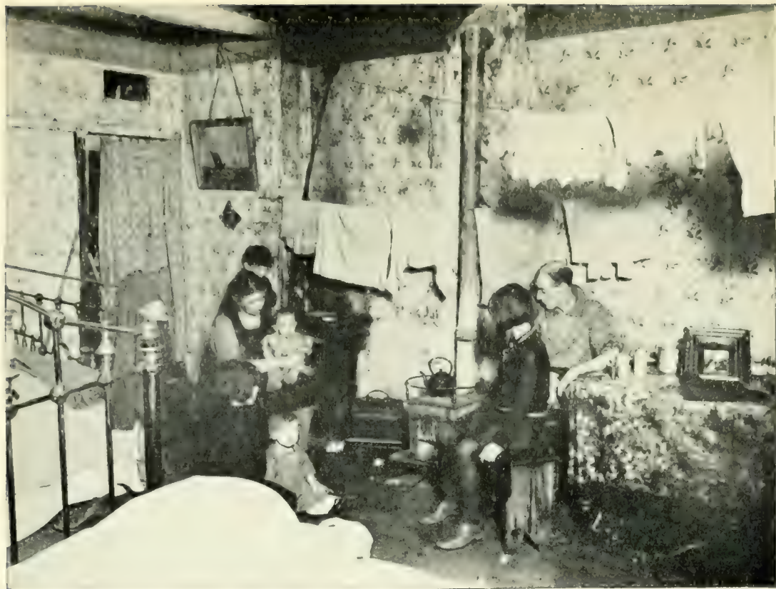
FIG. 64.—Interior of converted Warehouse used as a Dwelling-house, taken in a Northern Industrial Town in 1933.
