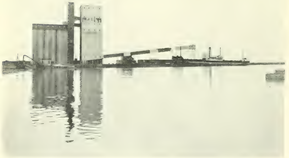
FIG. 47.—Loading the Wheat from the Elevator to Ship.
