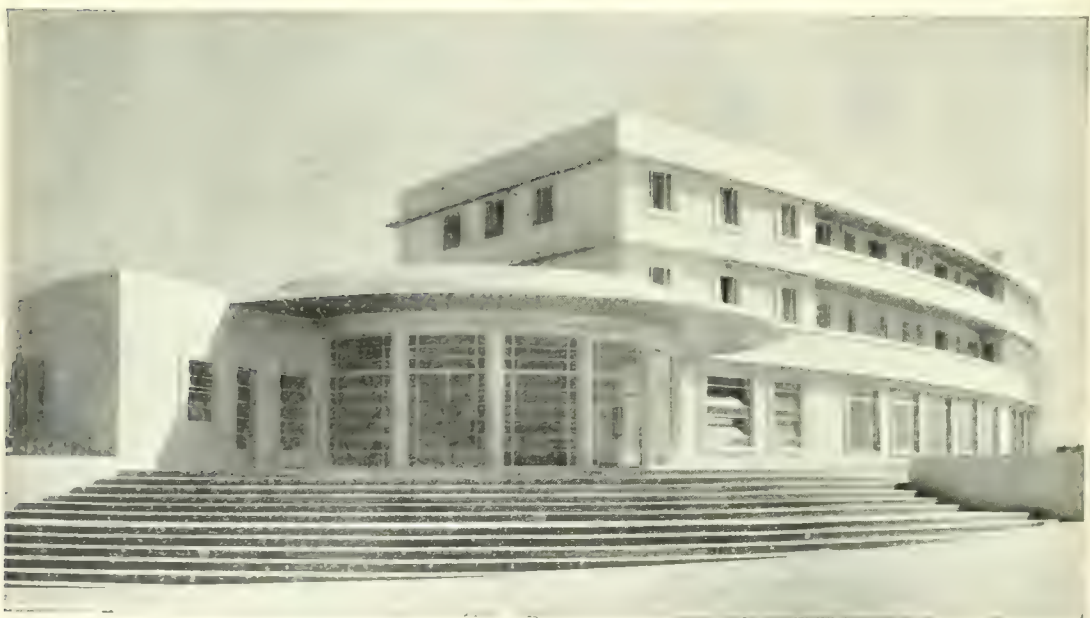
FIG. 129.—The L.M.S. Hotel, Morecambe, 1933. (Oliver Hill, Architect) [By courtesy of London, Midland & Scottish Railway Company.]
