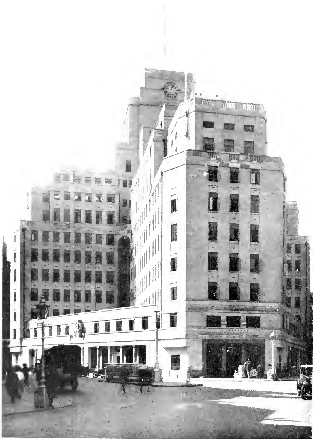
FIG. 120. The Underground Railway Offices at 55 Broadway, Westminster, London.
