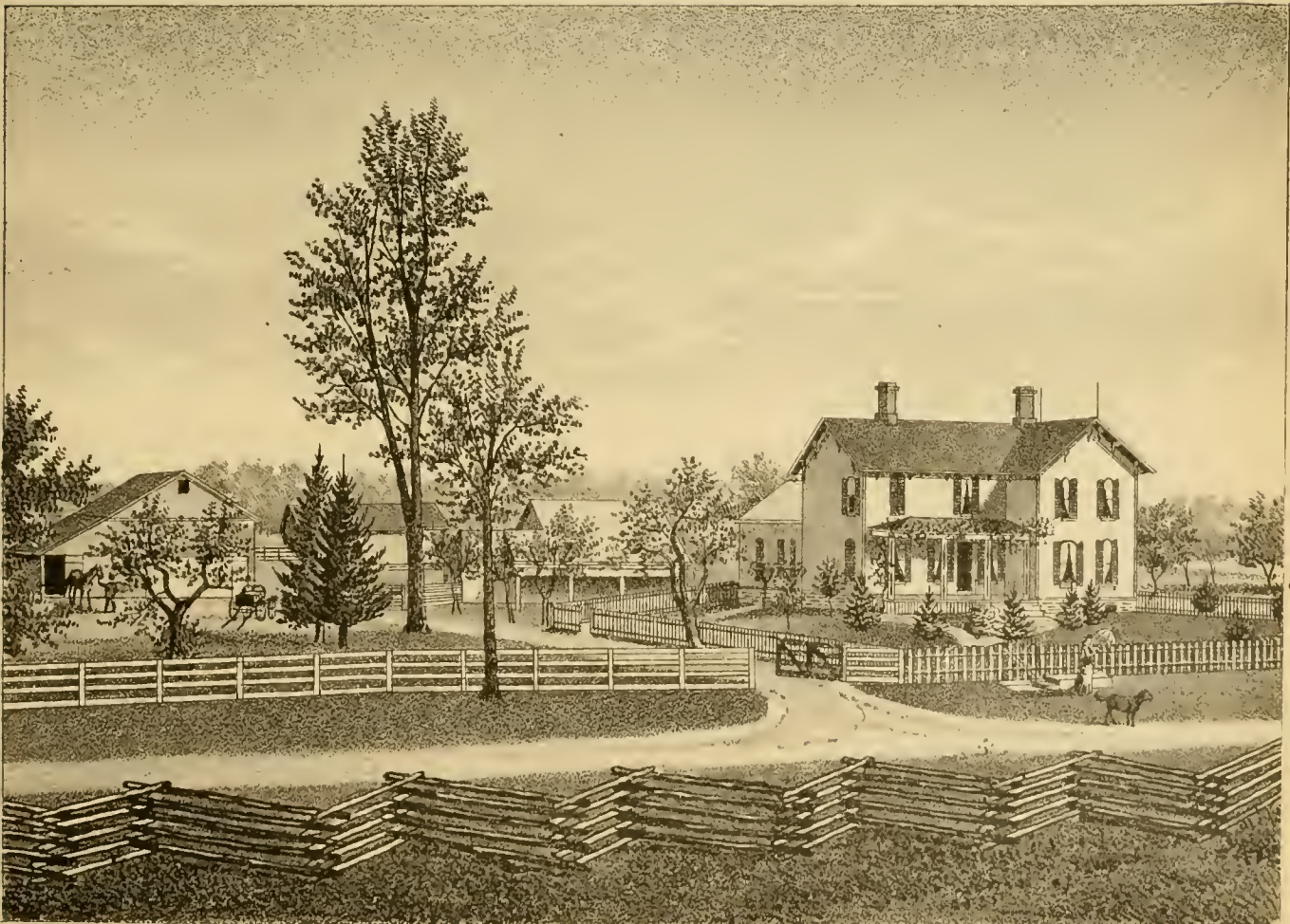
RESIDENCE OF A. J. BLACKMAN, CLARKSFIELD TP, HURON CO. O
