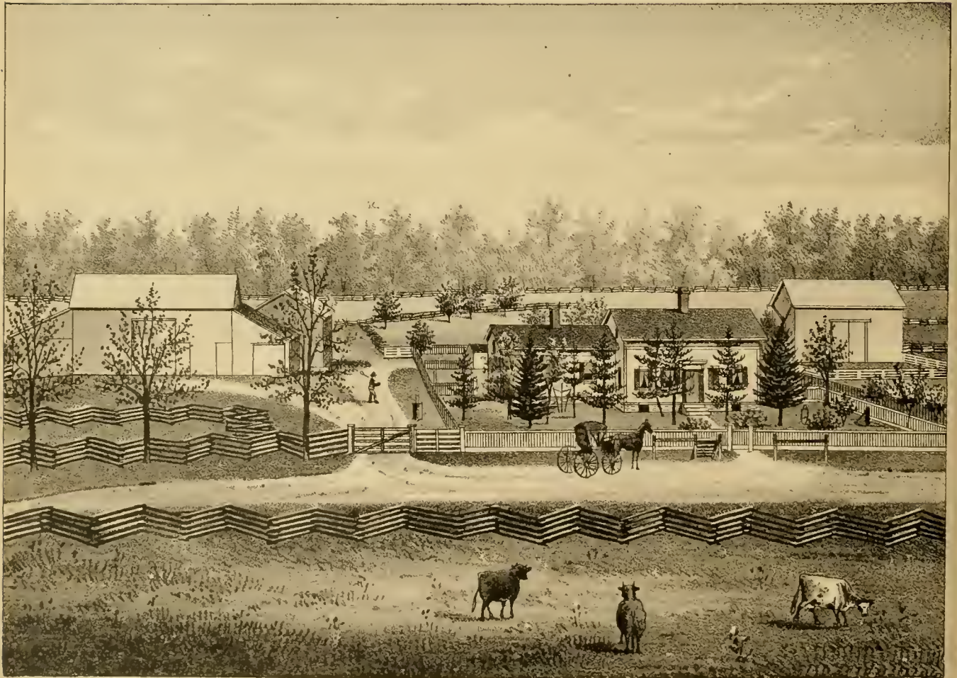
RESIDENCE OF JOHN S. HESTER, NORWICH Twp. HURON Co. O
