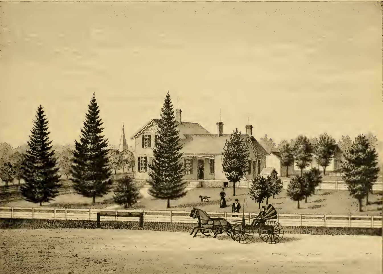
RESIDENCE OF R. G. RICHARDS, CHICAGO JUNCTION, HURON CO., O.
