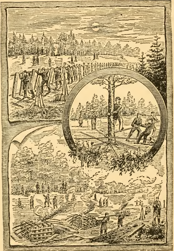
TEARING UP WELDON RAILROAD.
