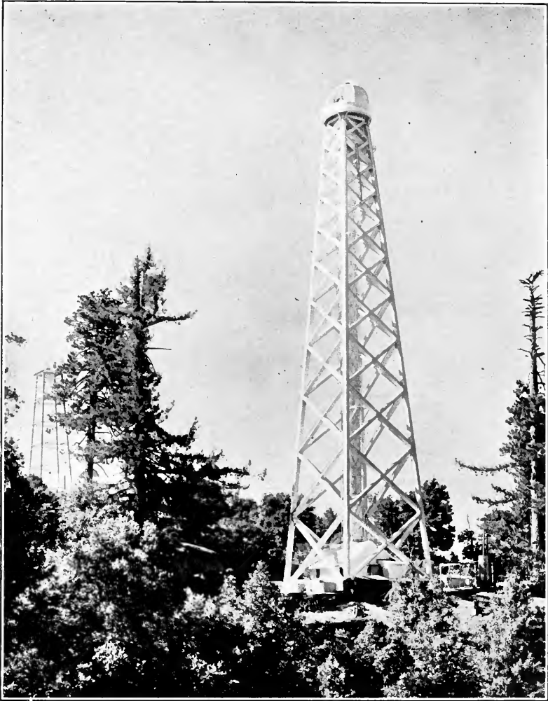
FIG. 13. 150-FOOT TOWER TELESCOPE.
