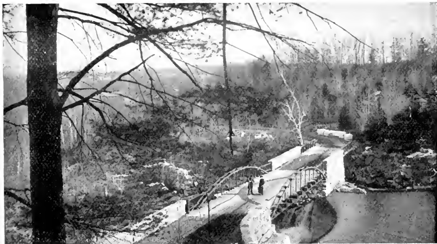
BRIDGE AT COOK'S DAM.
