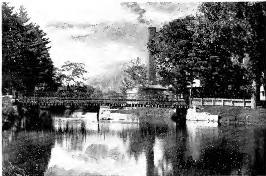
PINE STREET BRIDGE—A VISTA NEAR THE BRUSH FACTORY.
