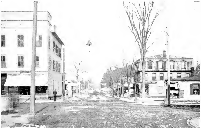
NORTH MAPLE STREET—FROM HOTEL CORNER.
