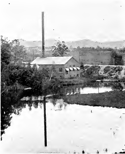
ELECTRIC POWER HOUSE—MOUNTAINS IN DISTANCE.
