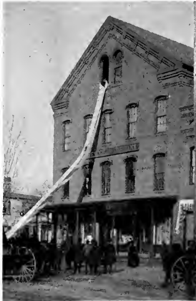
FIREMEN TESTING THE LIFE CHUTE.
