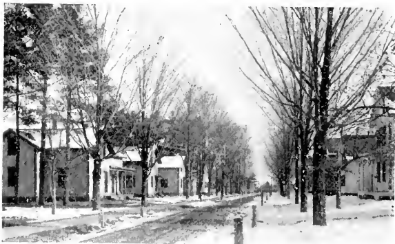
LOOKING EAST ON CENTER STREET.
