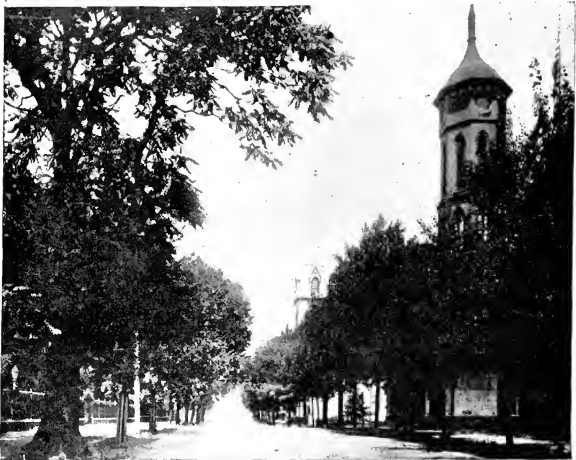
The Church and Signal Tower, Princess Anne Street, Fredericksburg.
