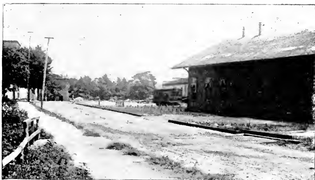
The Causeway over which the Regiment passed on its way to the charge.
