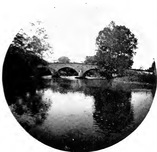
The Burnside Bridge in 1891.
