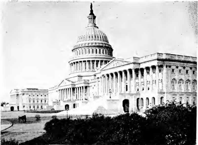
The Capitol, which was in process of rebuilding when the Fourteenth Regiment passed through Washington.
