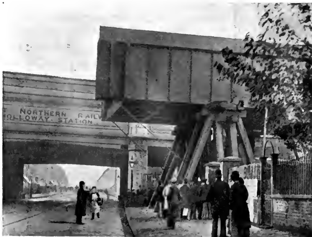
BRIDGE OVER HOLLOWAY ROAD WHEN IN COURSE OF DUPLICATION.
