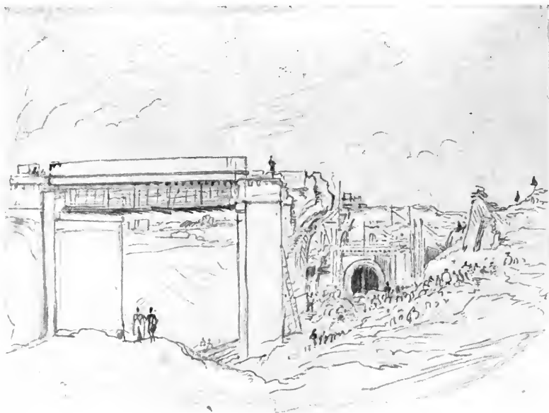
COLLAPSE OF THE NORTH LONDON VIADUCT NEAR KING'S CROSS.
