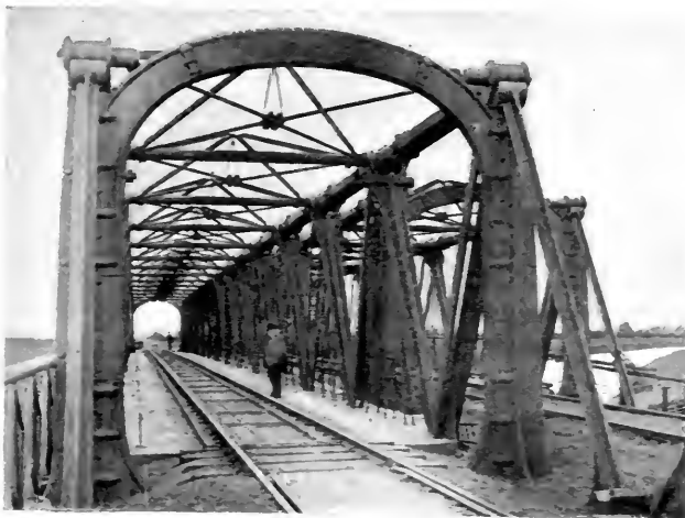
THE ORIGINAL "WARREN TRUSS" BRIDGE OVER THE TRENT NAVIGATION NEAR NEWARK.
