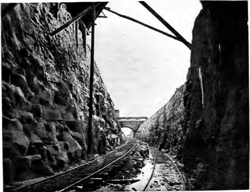
STRINES CUTTING, OVENDEN, NEAR HALIFAX, WHEN IN COURSE OF CONSTRUCTION.
