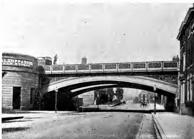
BRIDGE OVER FRIAR GATE, DERBY.
