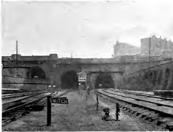
COPENHAGEN TUNNELS, KING'S CROSS (SOUTH END).
