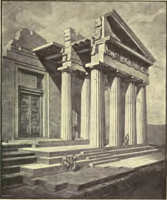
FIG. 56.—EAST FRONT OF THE PARTHENON, RESTORED AND DISSECTED. (From the Wiener Vorlegeblätter .)
