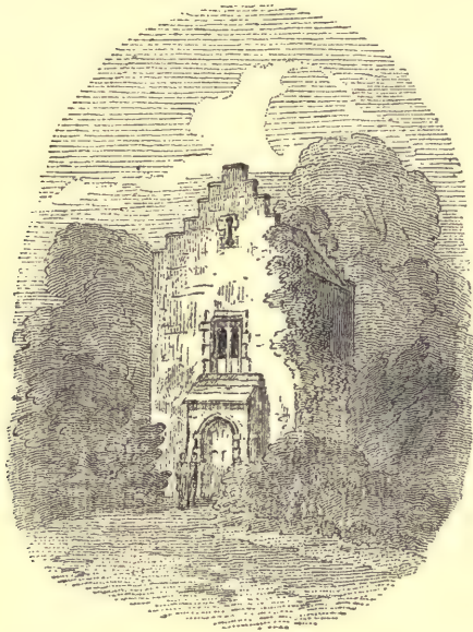
Water House at Coombe.
