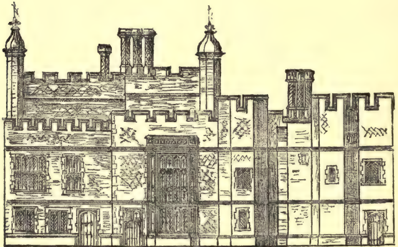
View of Cardinal Wolsey's Rooms in the Clock Court (now hidden by the Colonnade).
