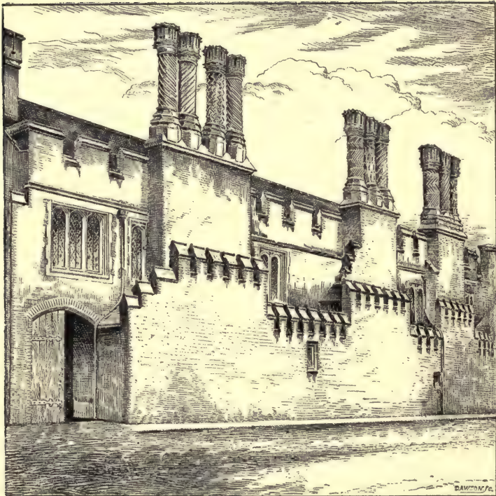
View of the Chimneys of the Great Kitchen, Tennis Court Lane.
