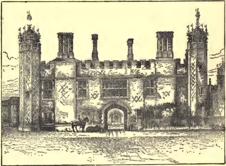
Entrance to the North Wing of the Palace, leading to the Offices.
