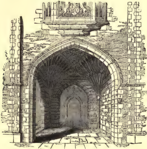
Foot of the Great Hall Stairs.
