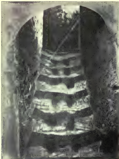
View from below of N.E. flight of rock-hewn steps—much worn. (Height of Arch, 6 ft. 2 in.)
