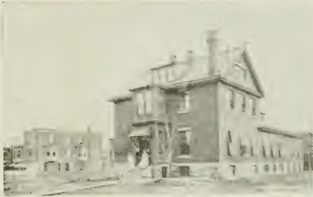
Sargent or Maternity Building.
