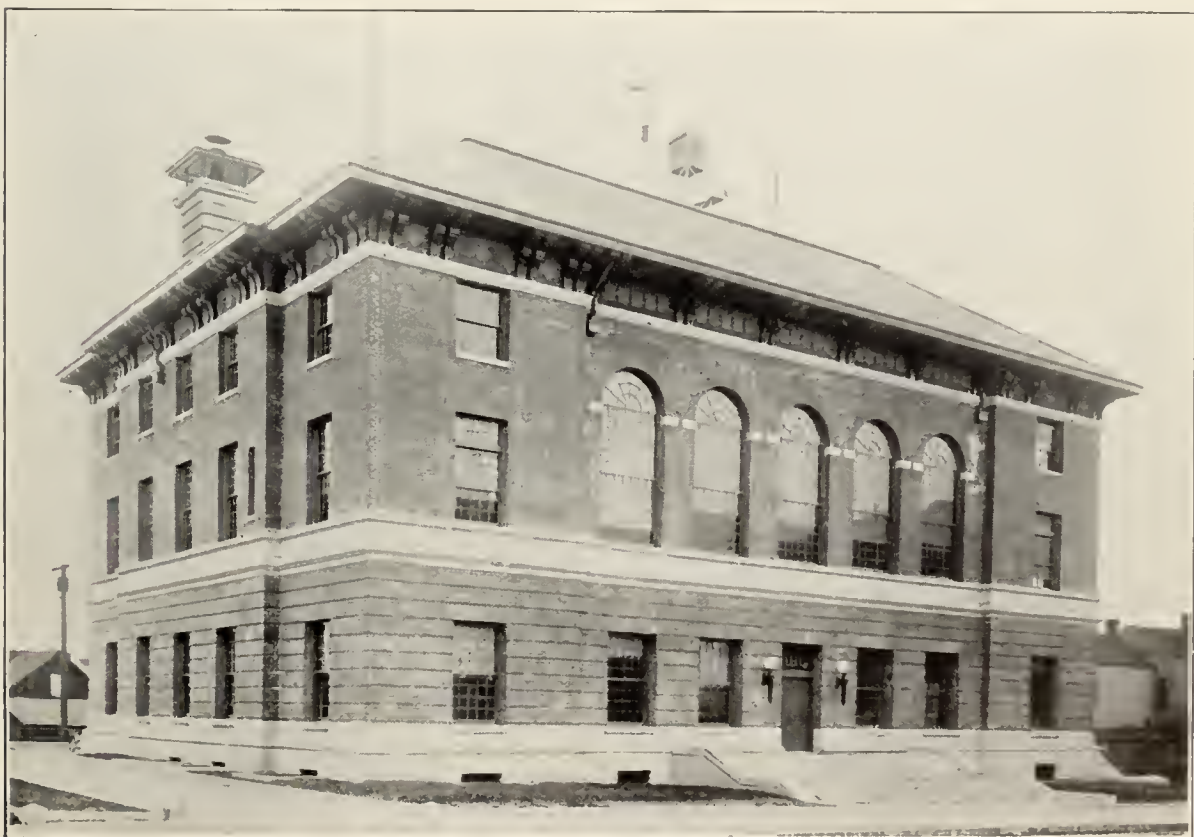
U. S. FEDERAL BUILDING AND POST OFFICE, EUREKA
