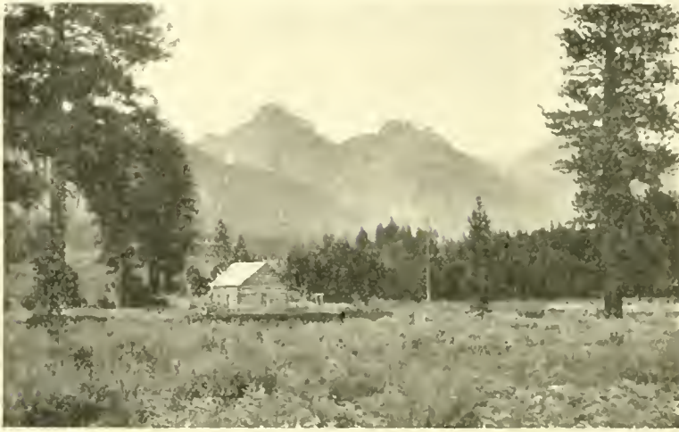
RANGERS STATION, IDAHO NATIONAL FOREST
