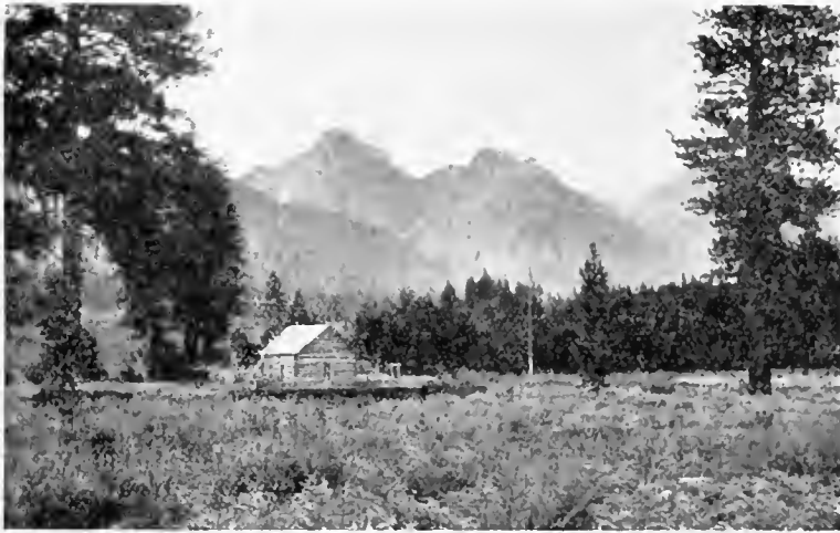
RANGERS STATION, IDAHO NATIONAL FOREST
