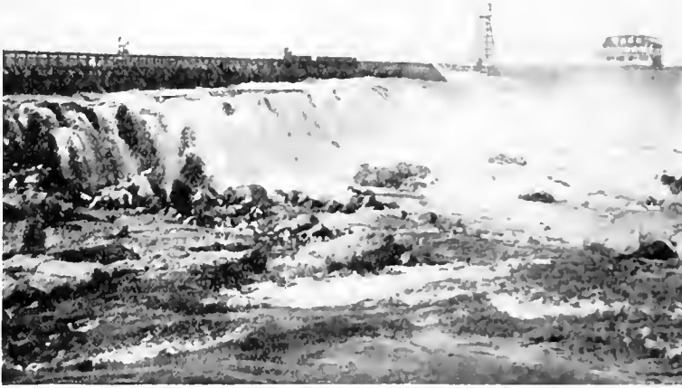
MILNER DAM, TWIN FALLS COUNTY
