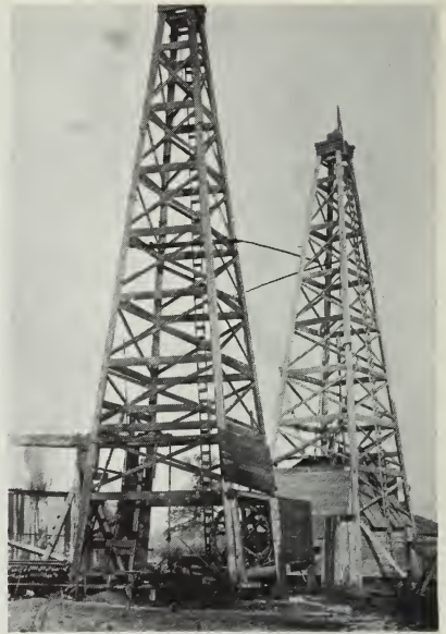
Wooden oil derricks operating in southeastern Illinois in the early 1900s.
