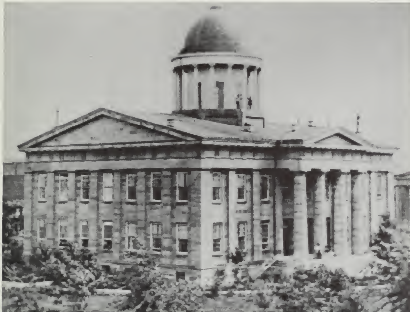
Fifth State Capitol Building built between 1837 and 1853 in Springfield, using local stone quarried at Crow's Mill, 7 miles south of town. The quarry site is now buried under Lake Springfield. (Photograph courtesy of Illinois State Historical Library.)
