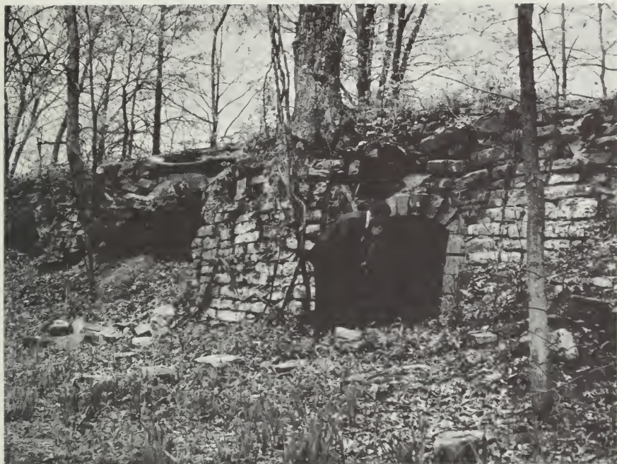
"Beehive" ovens located 2\frac{1}{2} miles southeast of Sparta in Randolph County. These ovens were used to convert Illinois coal to coke; operated in the 1880s.
