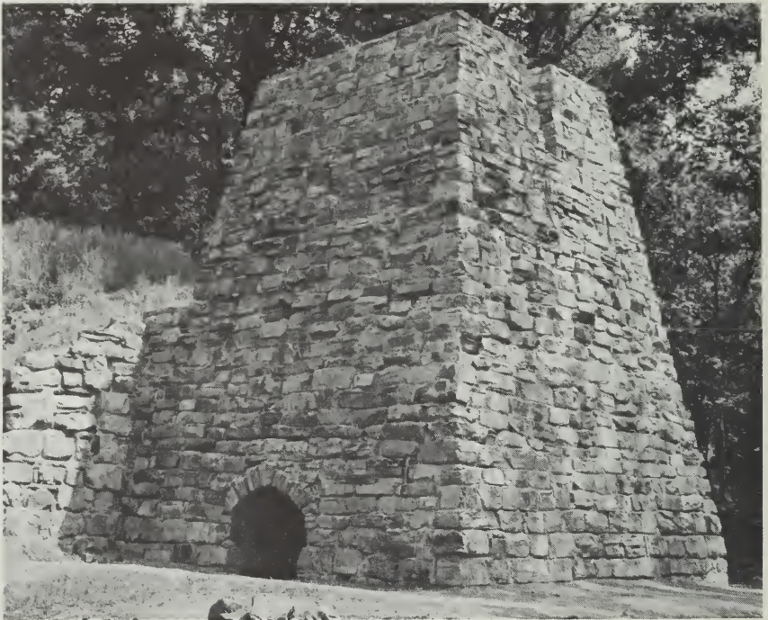
Illinois Furnace (1837 to 1883), first iron furnace in the state. Local iron ore was used in the furnace and charcoal was used for fuel. This furnace was reconstructed during 1966 and 1967. (Photograph courtesy of U. S. Forest Service.)
