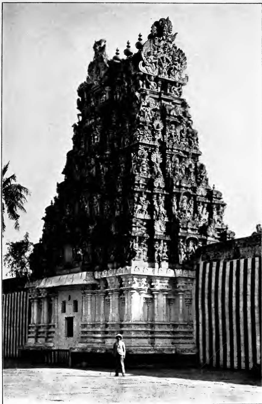
Smaller Gopura in West Court, Madurai. From a Photograph.
