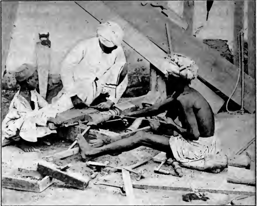
INDIAN CARPENTERS AT WORK.
