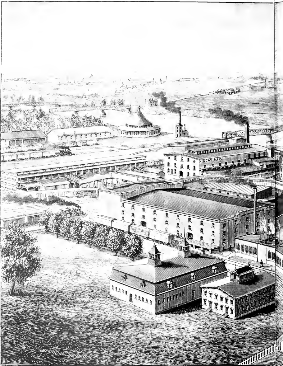
Morris Street Bridge,
