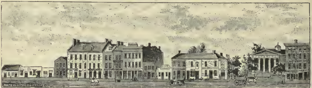
SOUTH SIDE OF WASHINGTON BETWEEN PENNSYLVANIA AND DELAWARE STREETS, 1848.
