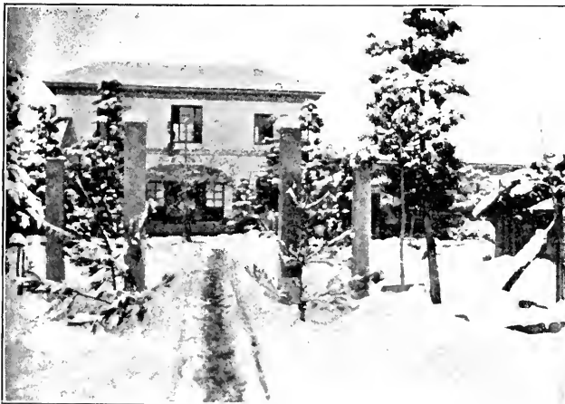
ENGLISH-JAPANESE SCHOOL BUILDING AS IT NOW LOOKS
