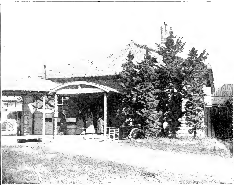
TEMPORARY QUARTERS, MIYAGI GIRLS' SCHOOL.
