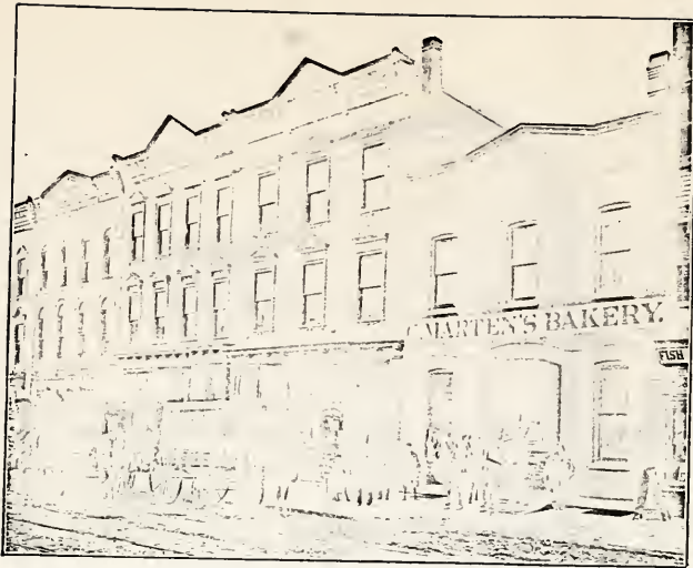
BUILDINGS OF C. MARTEN'S BAKERY.
