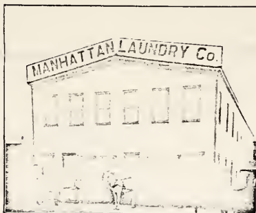
MANHATTAN LAUNDRY CO. BUILDING.
