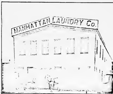
MANHATTAN LAUNDRY CO. BUILDING.
