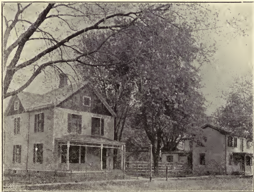
OFFICE AND HOSPITAL.
