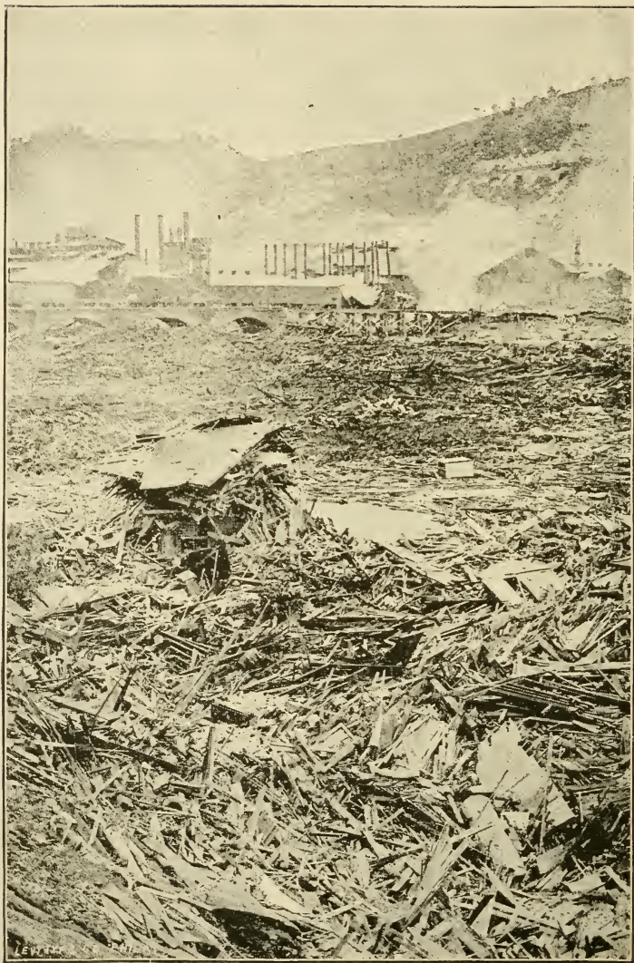
THE DÉBRIS ABOVE THE PENNSYLVANIA RAILROAD BRIDGE,
