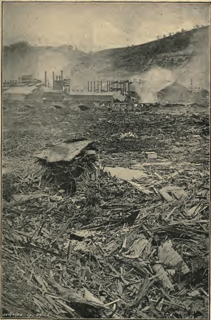
THE DÉBRIS ABOVE THE PENNSYLVANIA RAILROAD BRIDGE.
