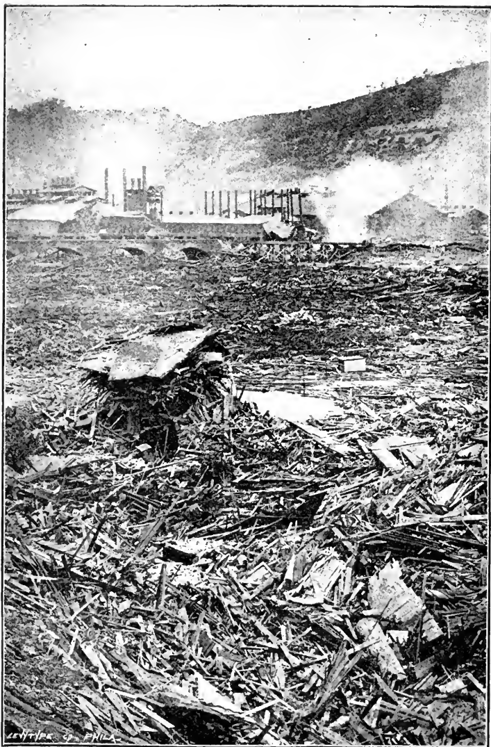
THE DÉBRIS ABOVE THE PENNSYLVANIA RAILROAD BRIDGE.
