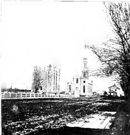
FIRST CONGREGATIONAL CHURCH AND CENTRE SCHOOL HOUSE, AURORA.
