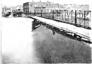
BRIDGE AT CHICAGO STREET, ELGIN.
