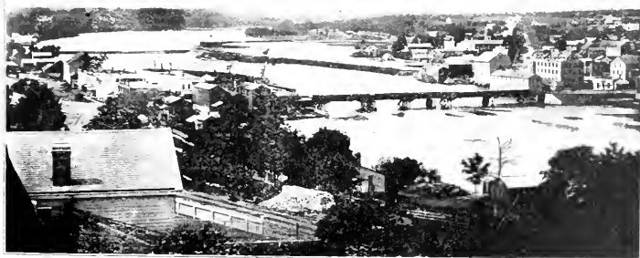
VIEW FROM BRIDGE NORTH—ELGIN—1866.
