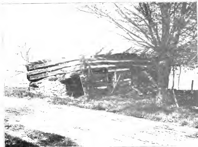
REMAINS OF A LOG CABIN STILL STANDING WEST OF ST. CHARLES.
