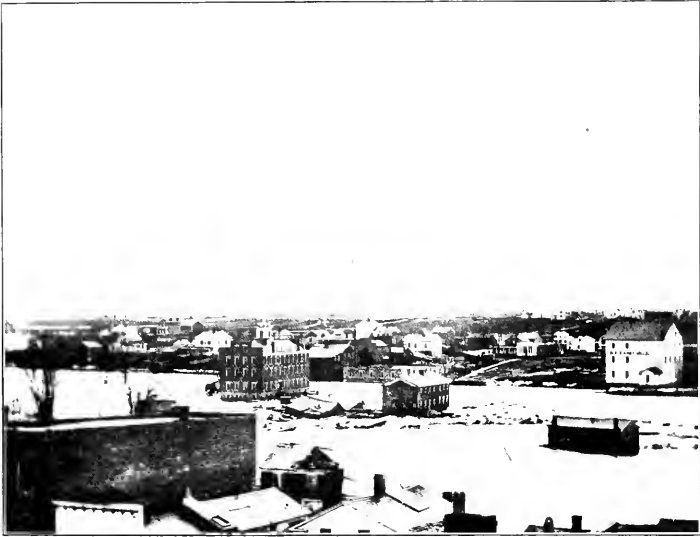
FLOOD OF 1857, AURORA, SHOWING SOUTH END OF STOLPS ISLAND.
