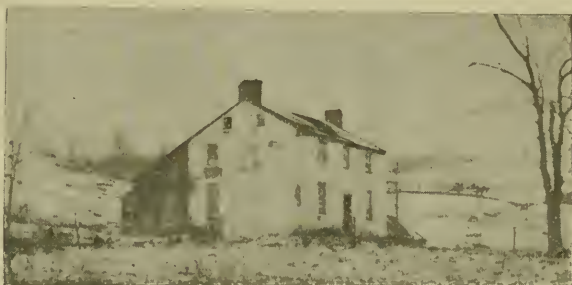
TOOL-HOUSE NOW STANDING NEAR THE OLD KENT IRON MINE.
