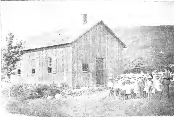
BULLS BRIDGE SCHOOL HOUSE.
