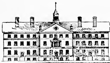
THE ORIGINAL COLLEGE BUILDING.
