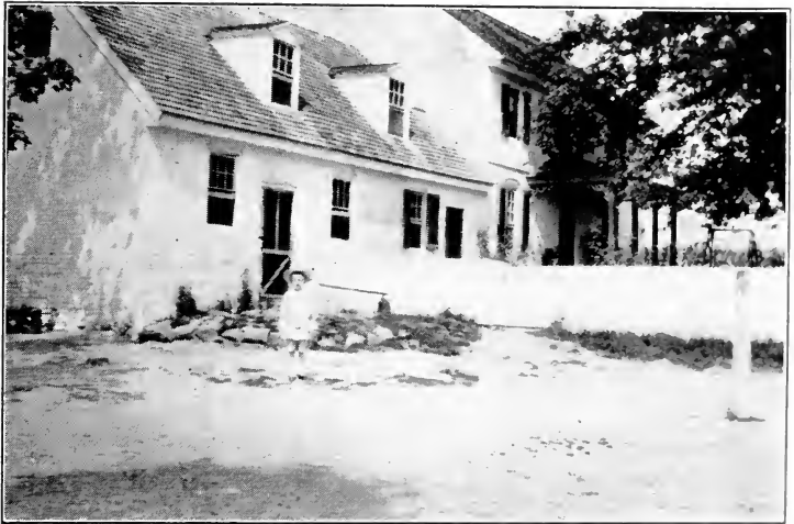
HOUSE BUILT IN 1687 ON "DUNCAN'S FOLLY," NEAR LYNCH. OWNED BY J. W. CHAPMAN AND OCCUPIED BY S. J. LEE.
